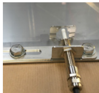
Figure 7 - Breakable burst sensor proper installation
